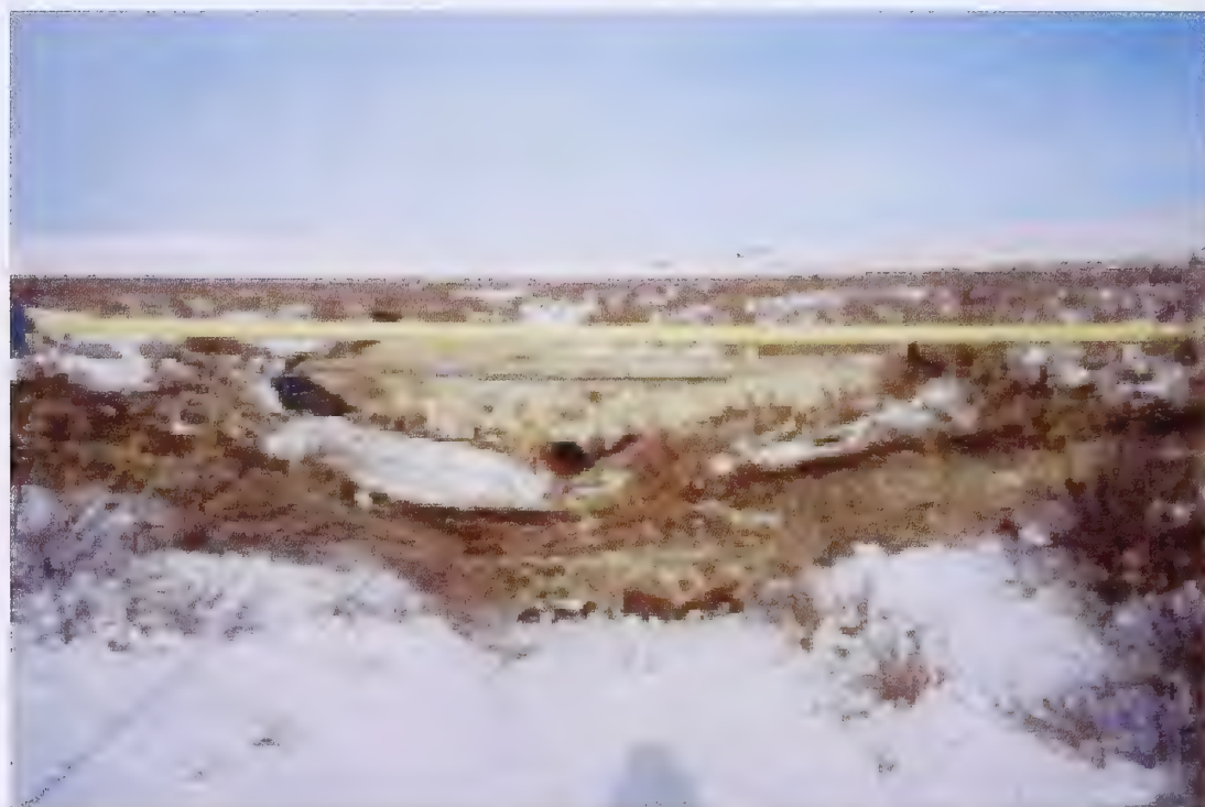
Photo 34 Woven geotextile used to facilitate the crossing of a seasonal drainage.
